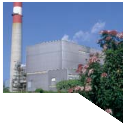
Barreiro thermoelectric power plant.
