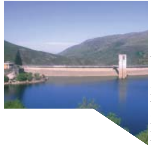
Vilarinho das Furnas hydroelectric power plant.
