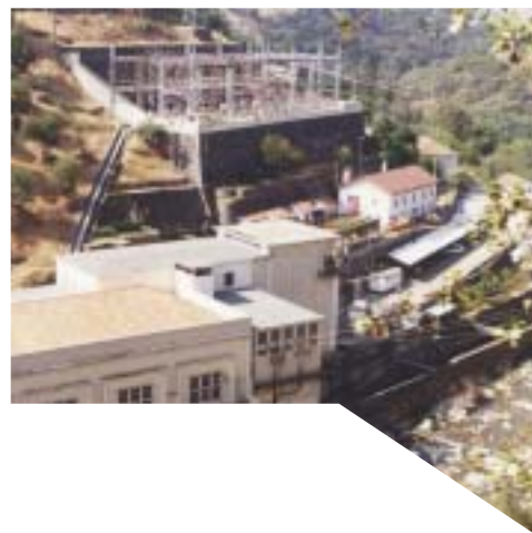
Varosa hydroelectric power plant.
