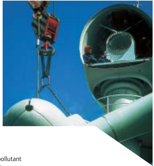
Fonte da Mesa – Installing wind turbine.
