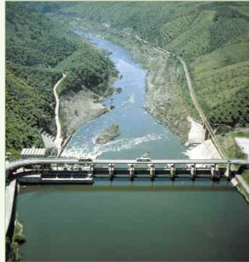
Fratel Hydro Power Plant
