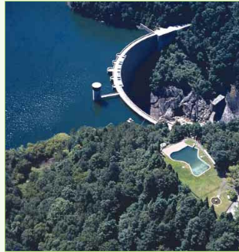
Caniçada Hydro Power Plant
